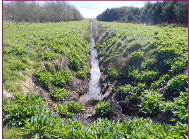
Photo 09: Example of the type of drainage channel.
