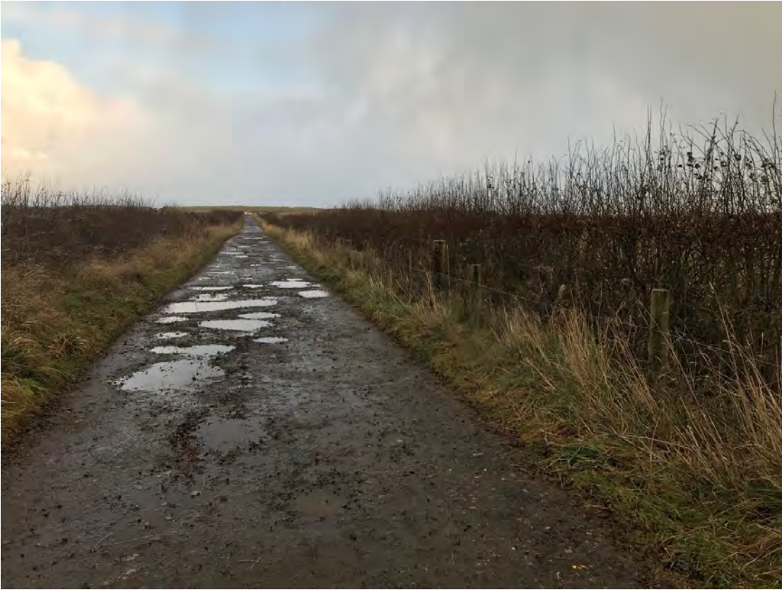
Plate 21: Typical view east along track to St Fergus' Church
